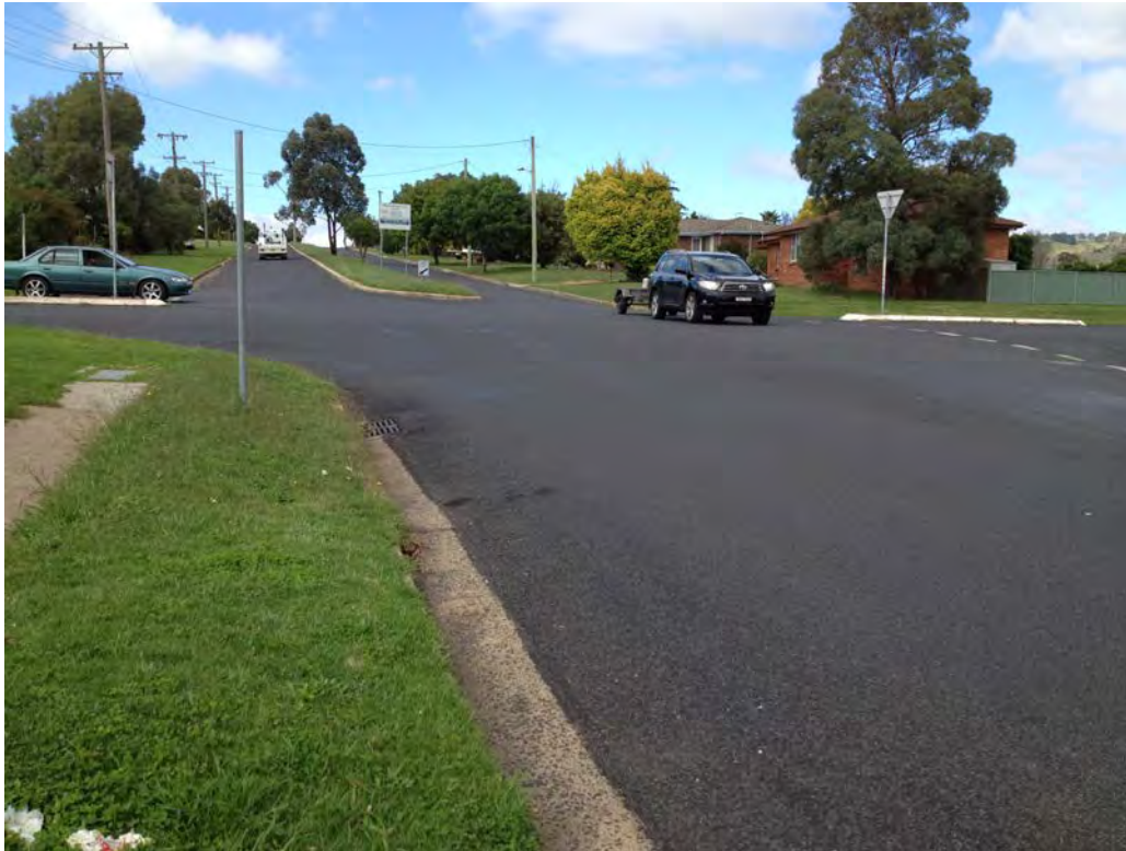
Plate 6 - College and Loyds Road Intersection looking south down College Road.
