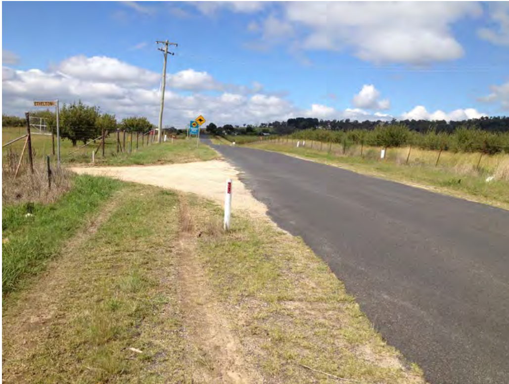
Plate 4 - College Road and Ethelton Avenue Intersection looking south towards the site.
