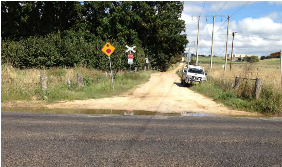
Figure 2: Ethelton Avenue railway crossing, looking west
